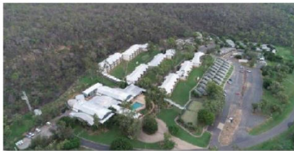
Dedicated accommodation village for over 400 workers
