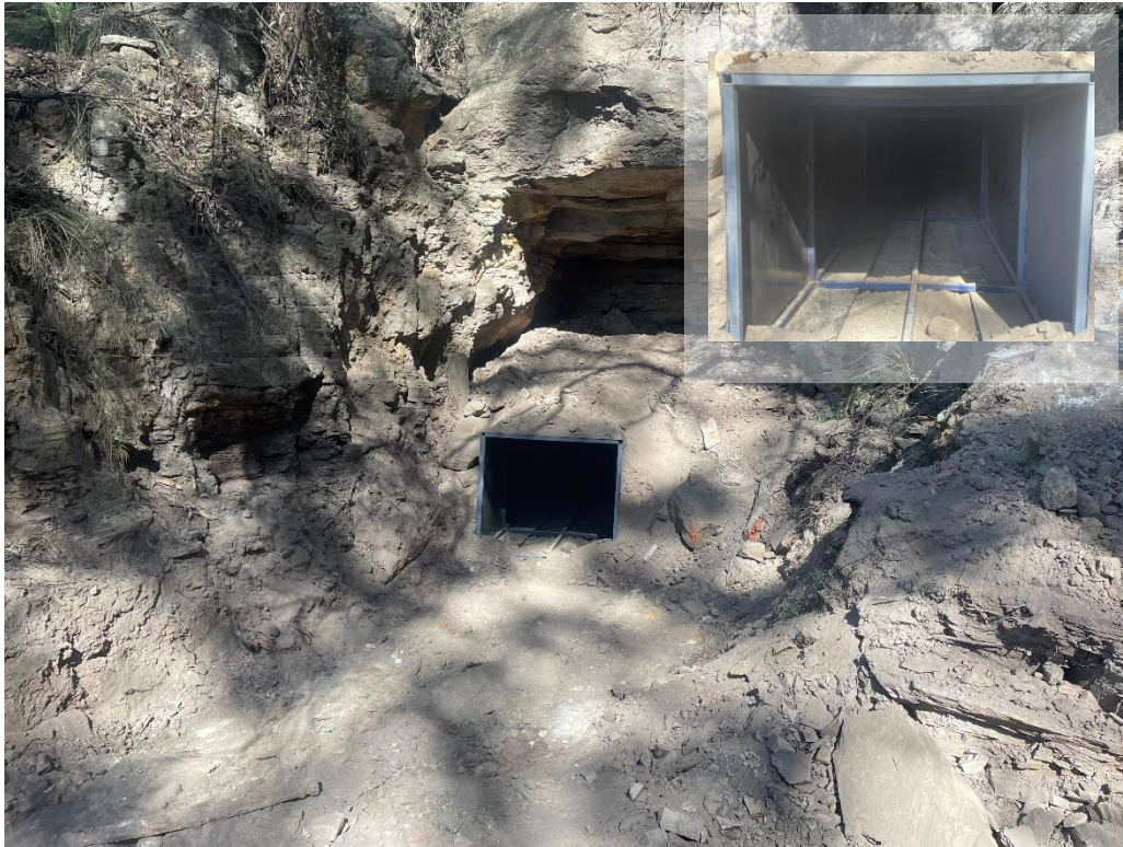
Photo 2 Upgrades in 2023 of the Culvert Entrance of the Mine Adit
