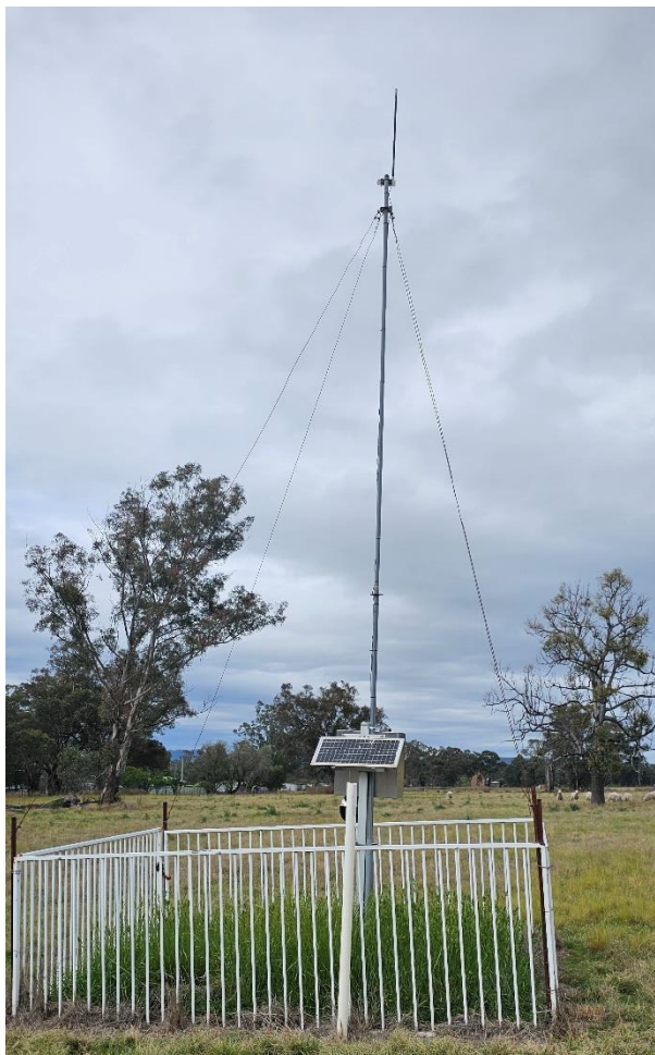
Plate 13 Fixed blast monitor at Wollar Public School
