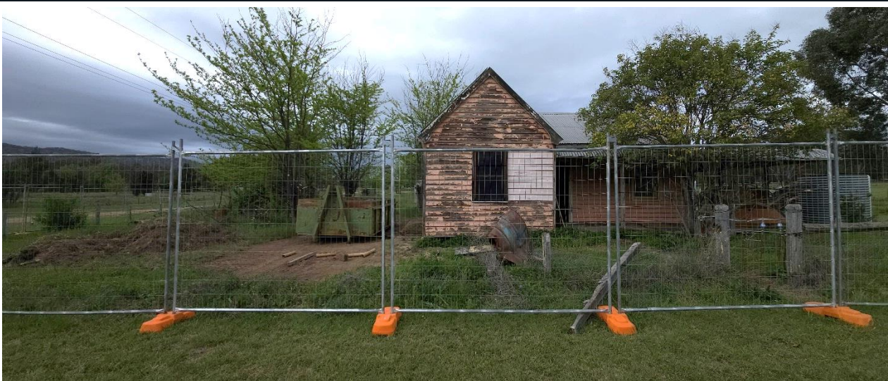
Plate 20 Derelict dwelling at Wollar Village to be demolished in the next IEA period
