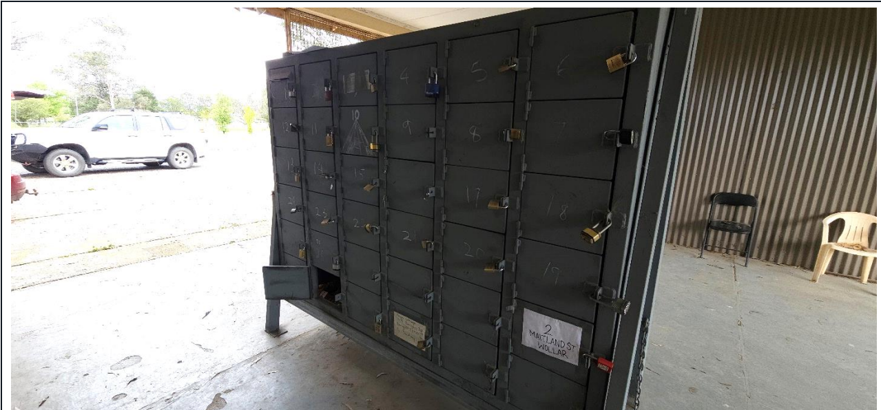
Plate 12 Replacement mailboxes provided by WCPL at former Wollar Store
