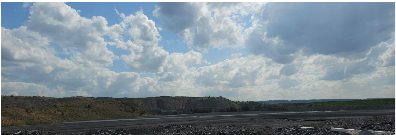
Plate 28 Operational tailings dam (TD6)
