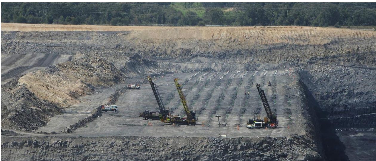
Plate 11 Blast drilling at Pit 6, facing north
