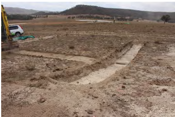
Plate 19: View looking east at the start of excavation of Trench 2.
