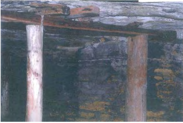
Plate 5: detail of wooden roof support structures (source: Niche 2015).
