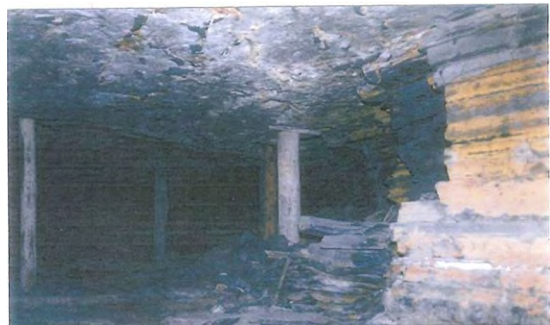
Plate 4: Detail of mine supports and face of shale deposit (source: Niche 2015).
