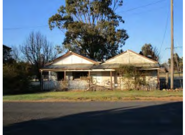
Plate A2-10 Former Butcher and Garage, Wollar (Niche, 2015)
