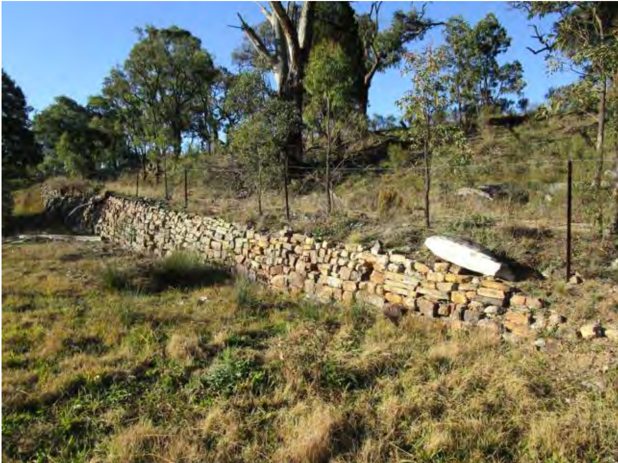
Plate 2 Road Embankment (Niche, 2015)
