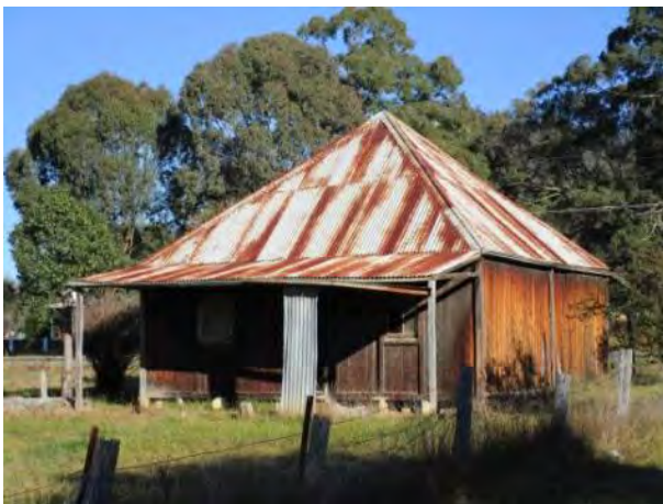
Plate A2-15 Slab Hut, Wollar (Niche, 2015)
