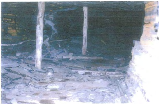
Plate 3: Interior of shale mine, showing wooden supports (source: Niche 2015).
