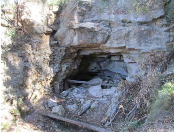
Plate 7: The mine adit (Niche, 2017)
