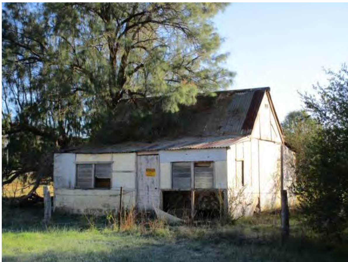
Plate 14: The original front facade and setting of Kirkland's Hut, prior to the tree falling on the structure (Source Niche 2015).
