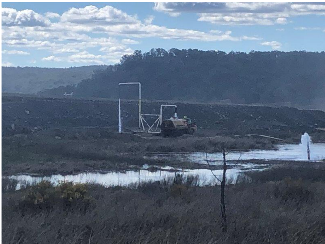
Plate 24 – Water cart being refilled during inspection
