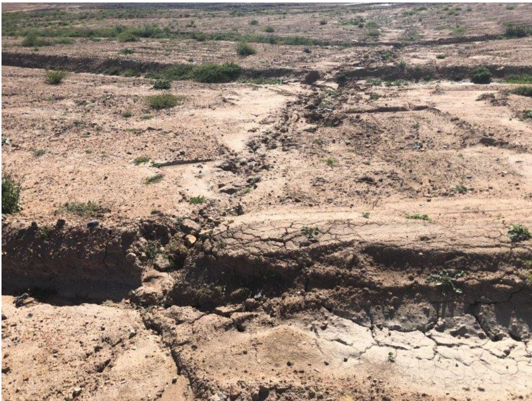
Plate 28 – Example of poor construction of graded bank leading to sedimentation and bank failure.
