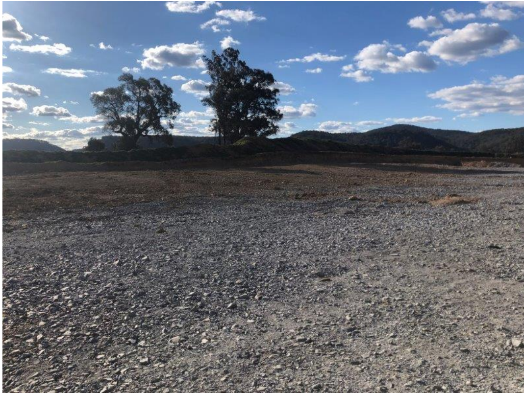
Plate 33 – Eastern tie in to Cumbo Creek
