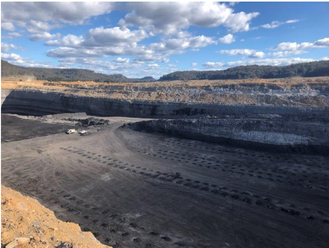
Plate 30 – Pit 8 shots drilled prior to blasting
