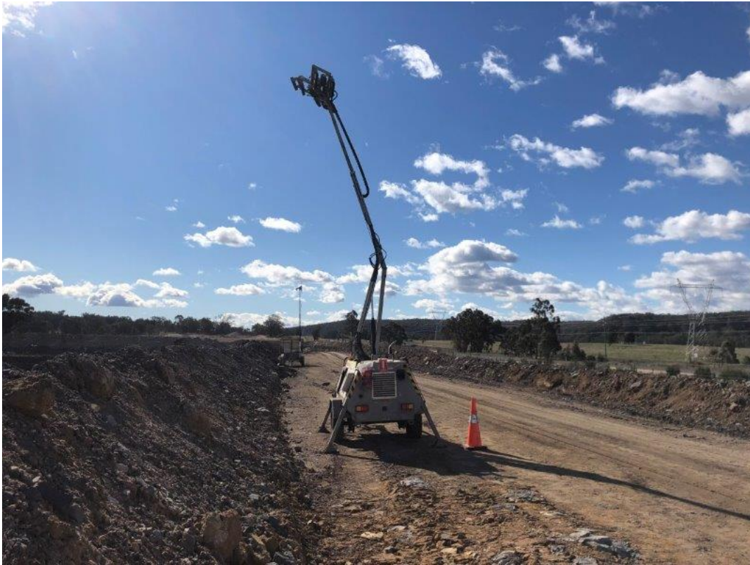
Plate 17 – Mobile lighting rig pointing into Pit 6
