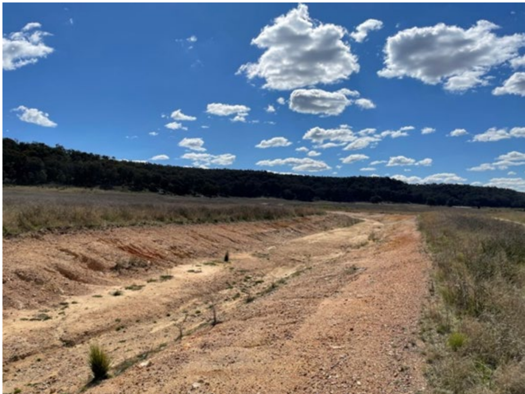
Plate 42 – Clean Water Diversion Pit 8
