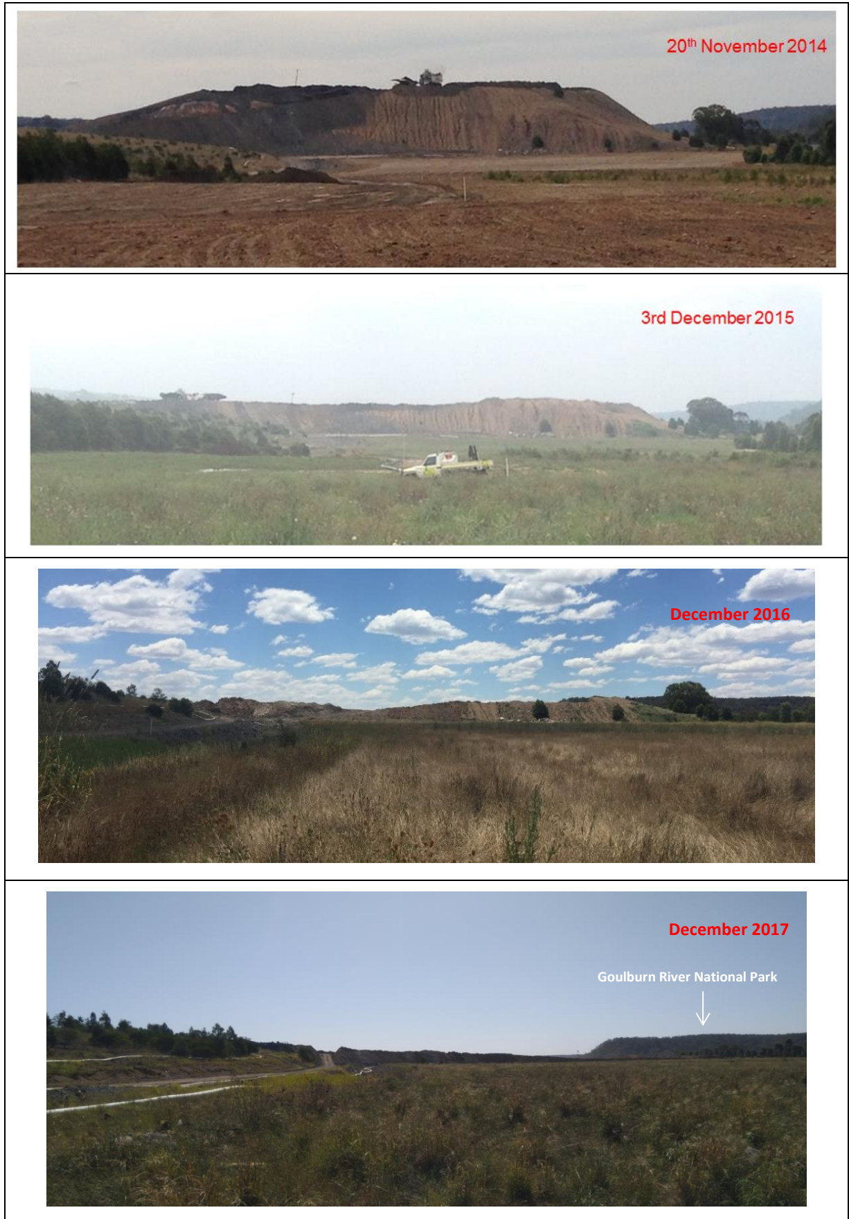
Figure 3 Completion of Keylah Dump Removal
