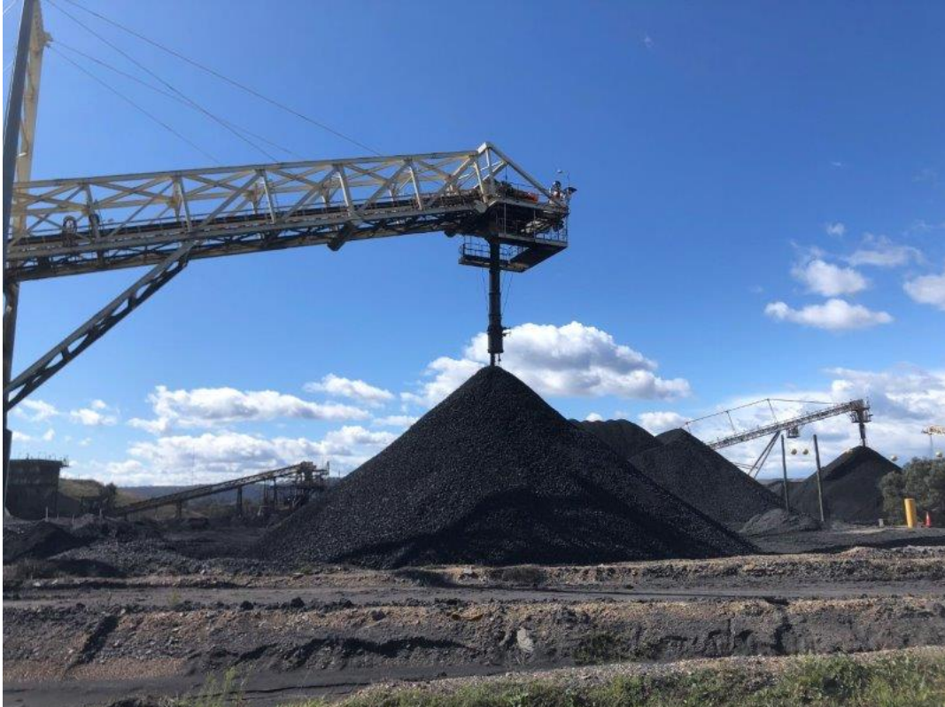
Plate 8 – Washed coal stockpile near CHPP
