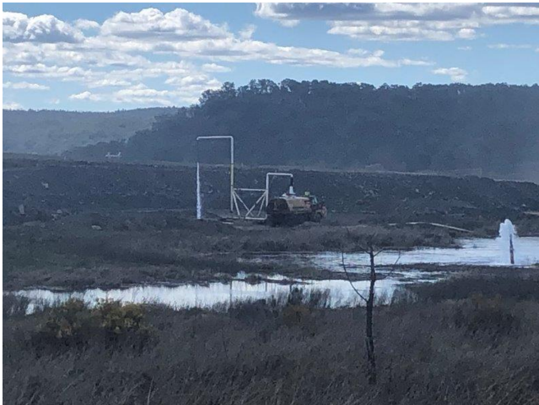
Plate 24 – Water cart being refilled during inspection
