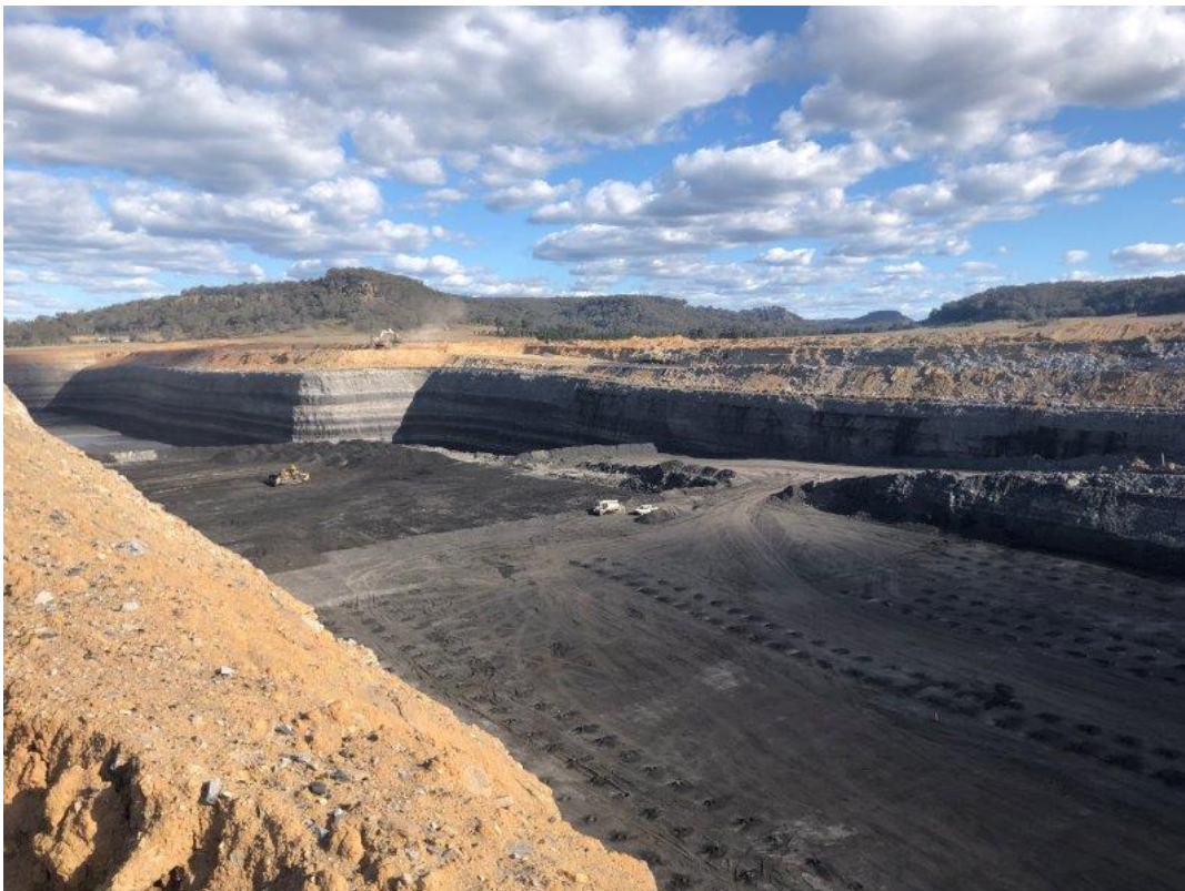
Plate 32 – Pit 8 shots drilled prior to blasting
