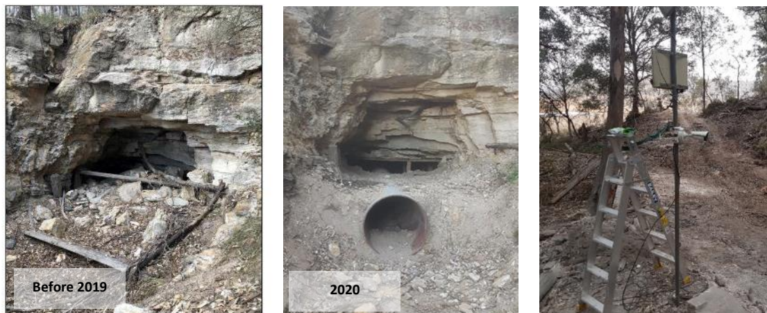
Photo 1 Culvert Support & Bat Detector with Solar Panel setup 20m in front of Adit
