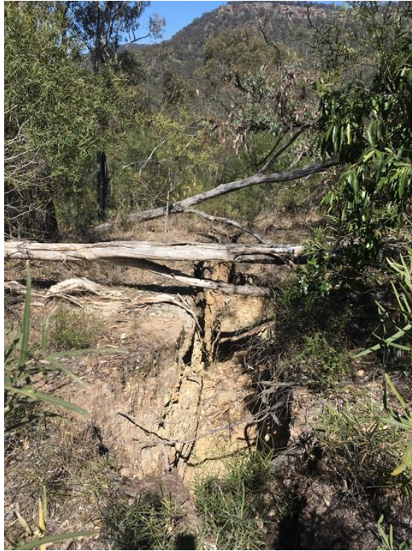
Plate 27: Deep mine subsidence cracks on ridgeline near bird monitoring site BP12
