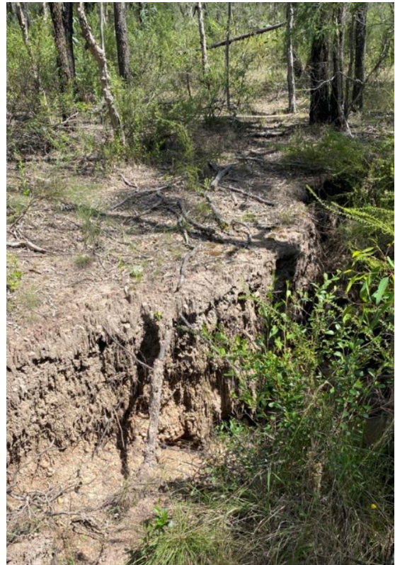
Photograph 38: Large subsidence cracks near flora monitoring site V11-B1 (in 2022)
