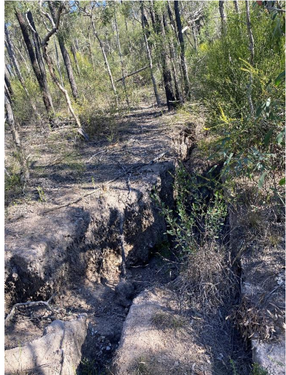
Photograph 40: Large subsidence cracks near flora monitoring site V11-B1 (in 2023)
