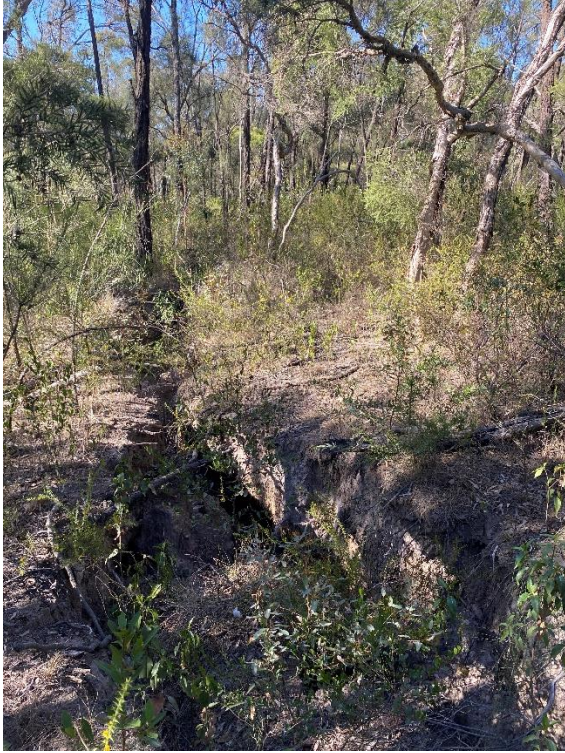
Photograph 39: Large subsidence cracks near flora monitoring site V11-B1 (in 2023)
