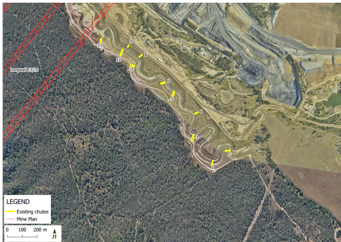
Figure 2. Location of existing batter chutes along both the downstream portion of NWCD and the portion over LW11-LW16
