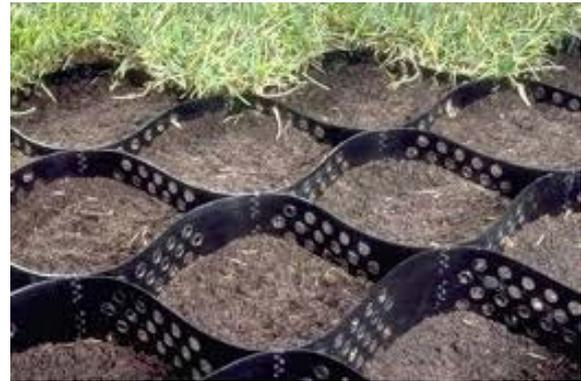
The use of this system as an erosion control device is discussed in more detail in Guideline H347052-0000-10-215-0010 Cellular Confinement Systems (Erosion Control).
