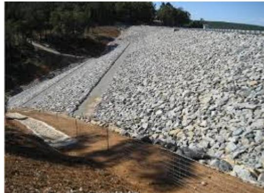
For rock lining in concentrated flow paths, refer to the drainage control "rock lining" guideline.
