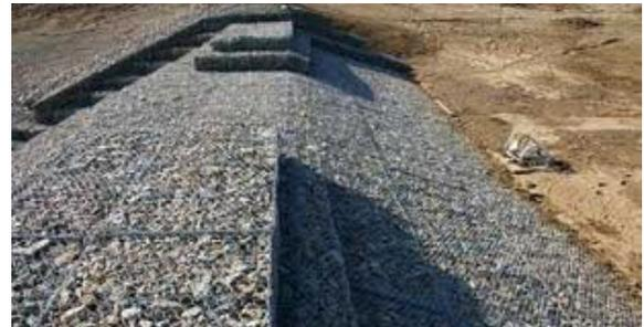
Mattresses are constructed on the ground and can be linked together to cover large surface areas. The rock fill provides the weight to resist shear flow and the wire cells aid in withstanding movement of the rock.
