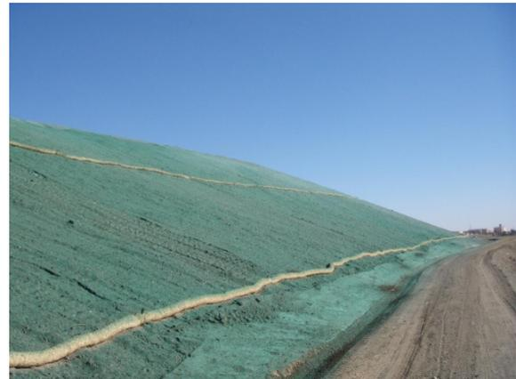
Soil binders can either be sprayed directly over an exposed surface or applied as tackifiers in conjunction with mulching and seeding applications.
