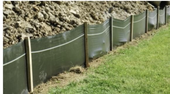
Sediment fences are created using special purpose synthetic material laid vertically by securing to stakes and anchored the toe of the fence in to a trench.
