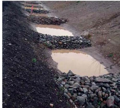
Check dams may also be used as a drainage control, and although the intended function is different, the design and construction methodology remains the same.
