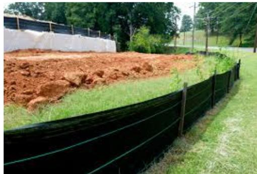
**Figure 9: Example of Sediment Fencing**
