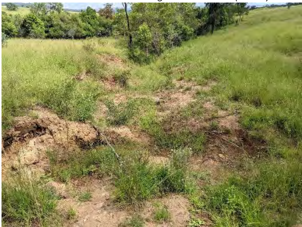
Waterfall Creek tributaries downstream of LW 25 & 26. Incised channel with some bed erosion (2022)
