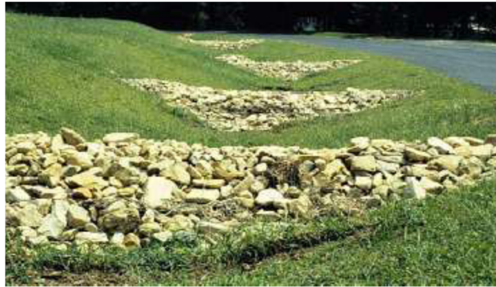
Figure 8: Example of Check Dams
