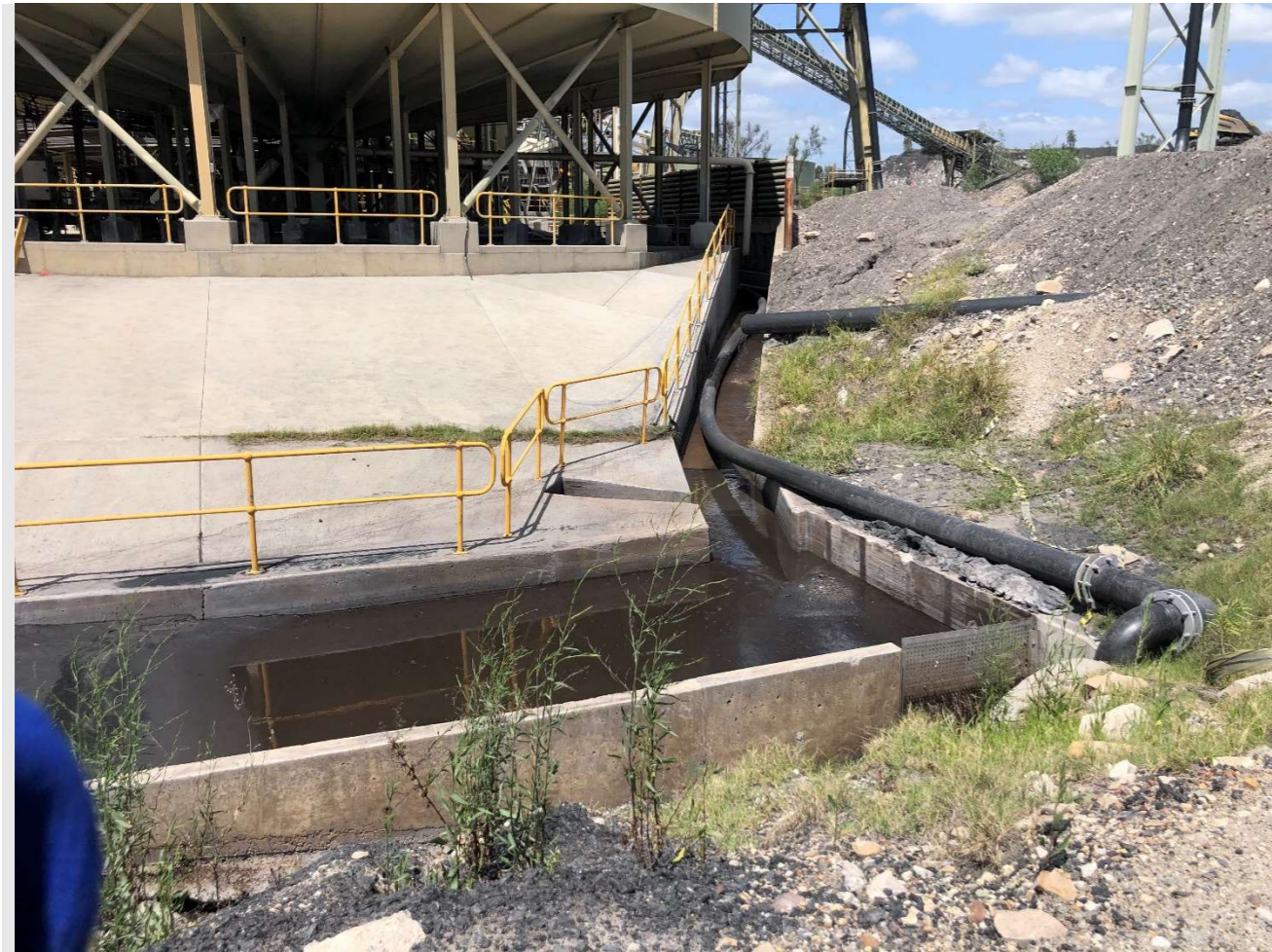
Plate 17 Coal contact flow path at CHPP
