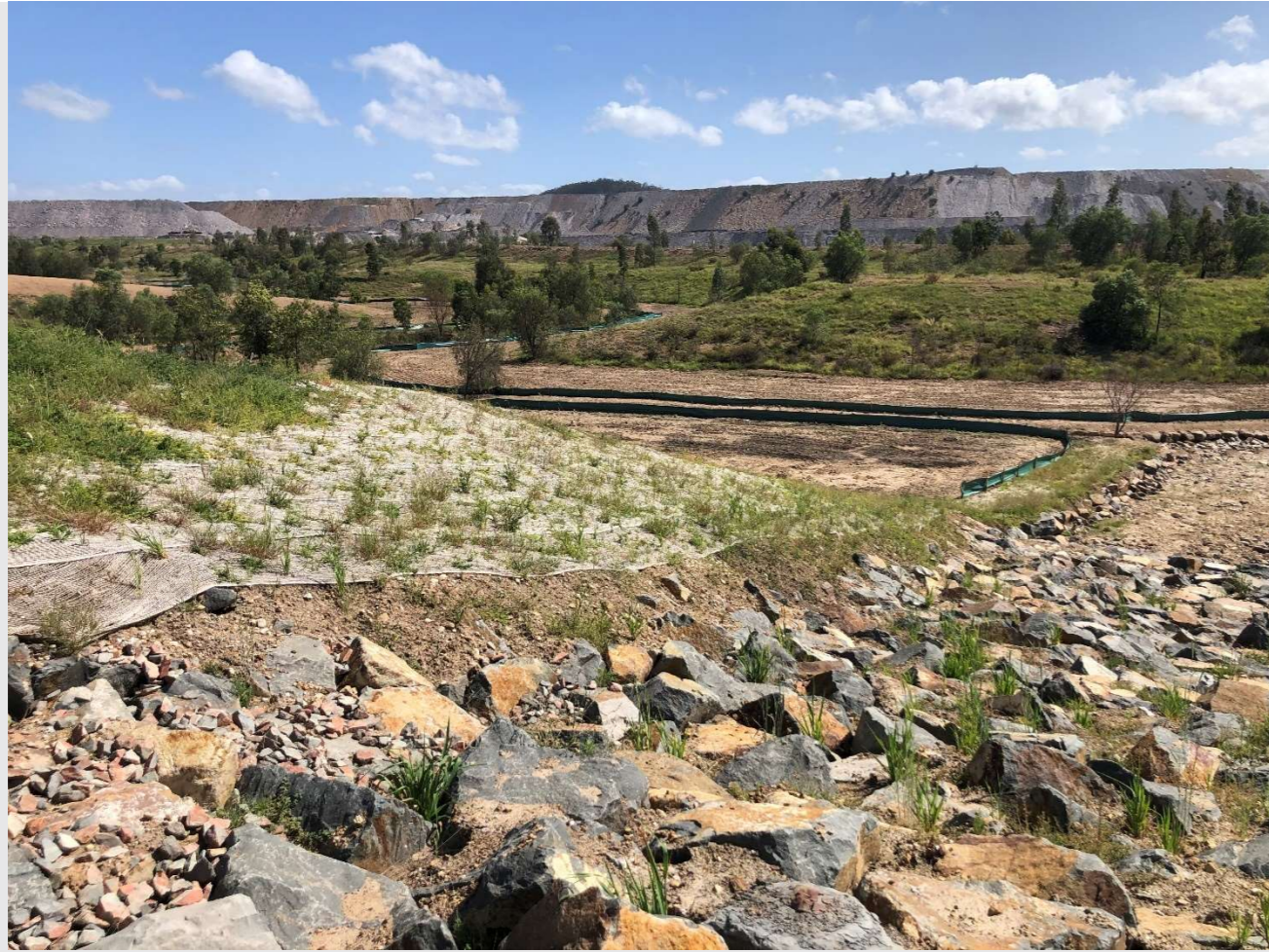
Plate 9 North Wambo Creek Diversion Rehabilitation Works
