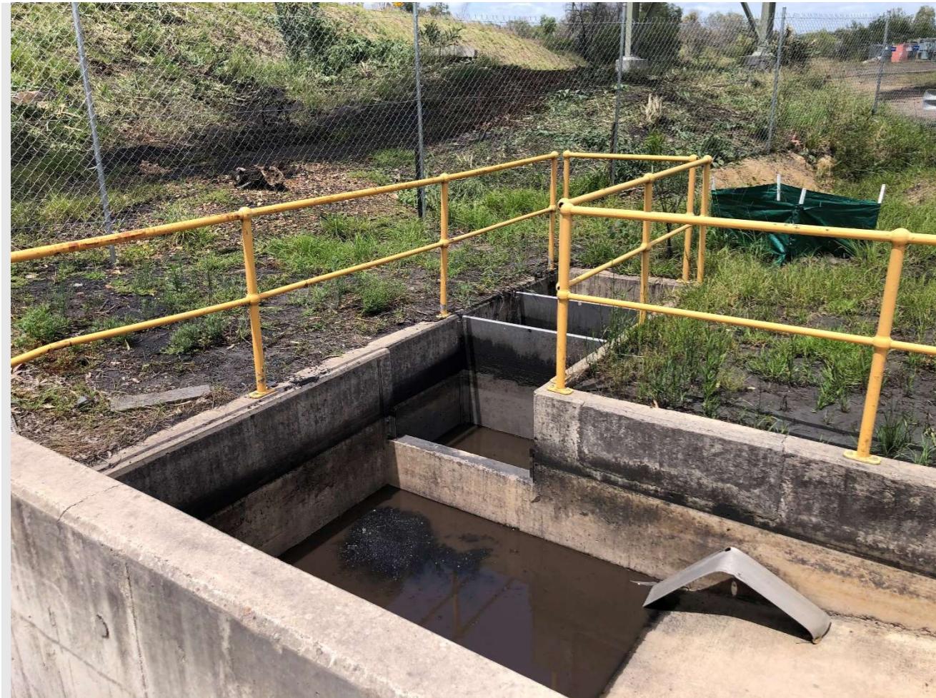
Plate 19 Upper Train Load Out Pad Sump
