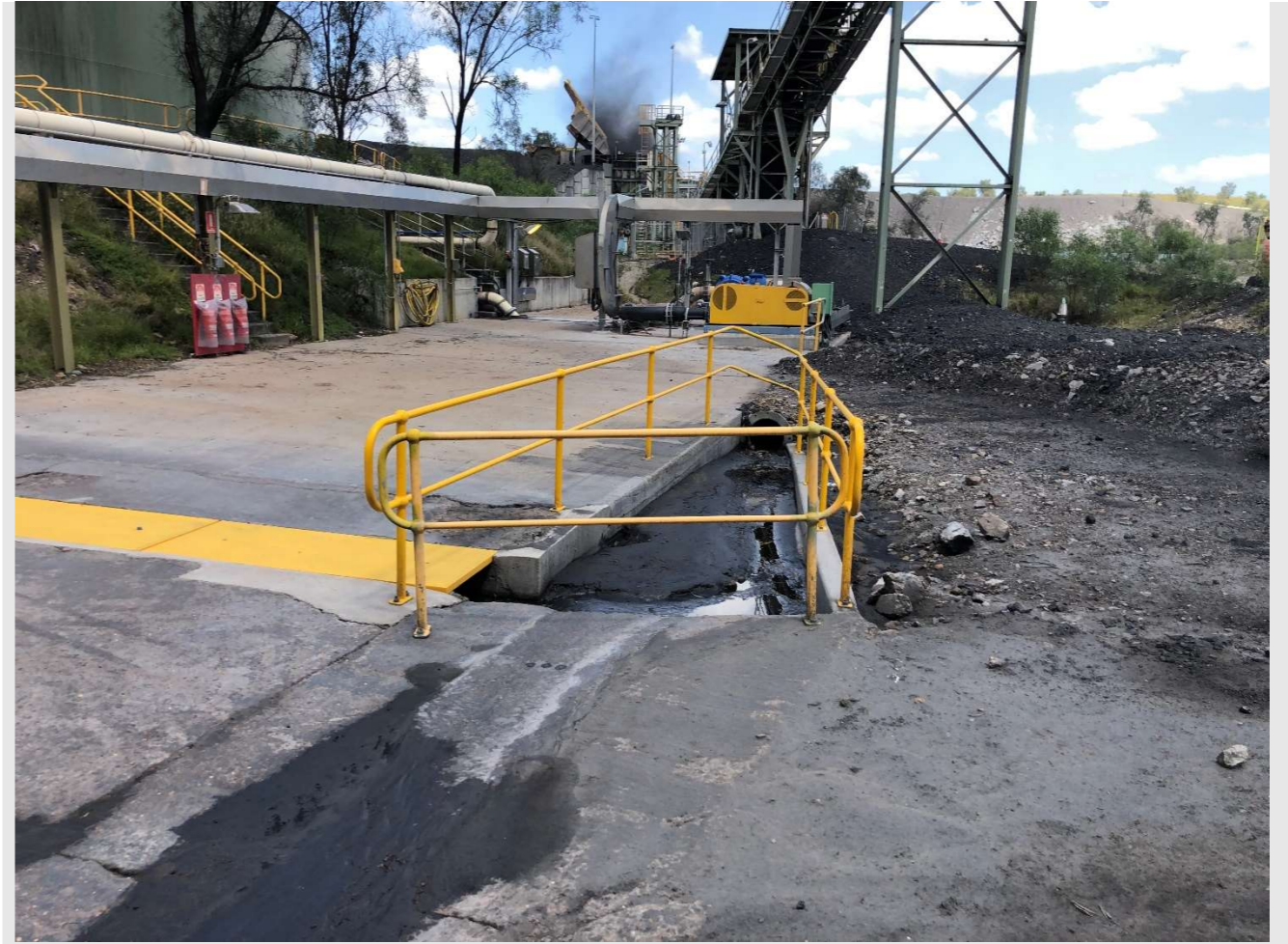
Plate 16 Coal contact flow path at CHPP
