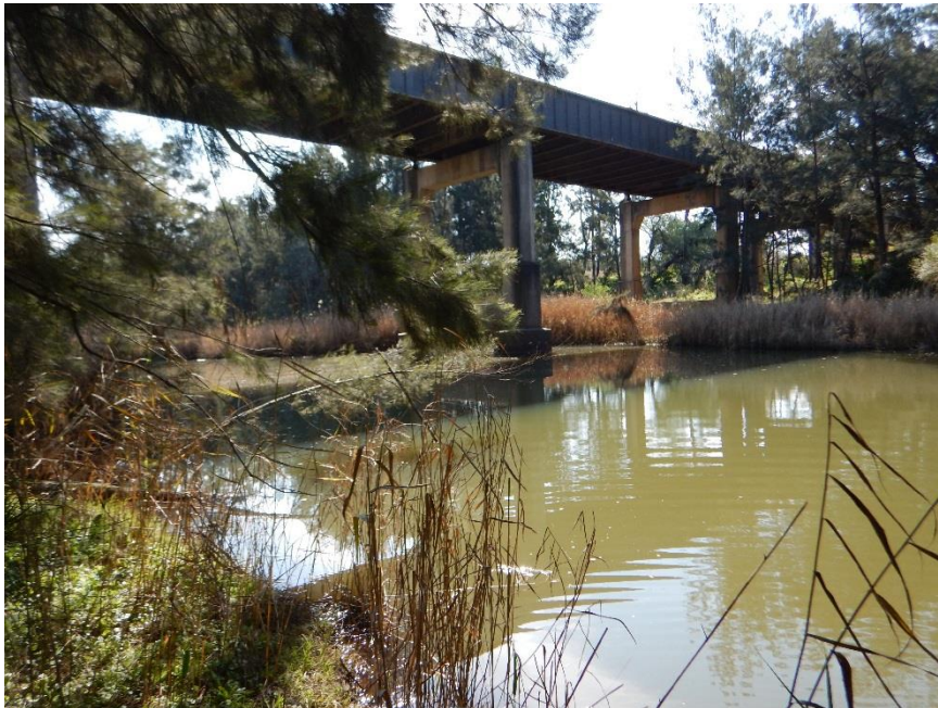
Plate 12 Site 10 Wollombi Brook at downstream bridge (Golden Highway) (314308E 6395036N)
