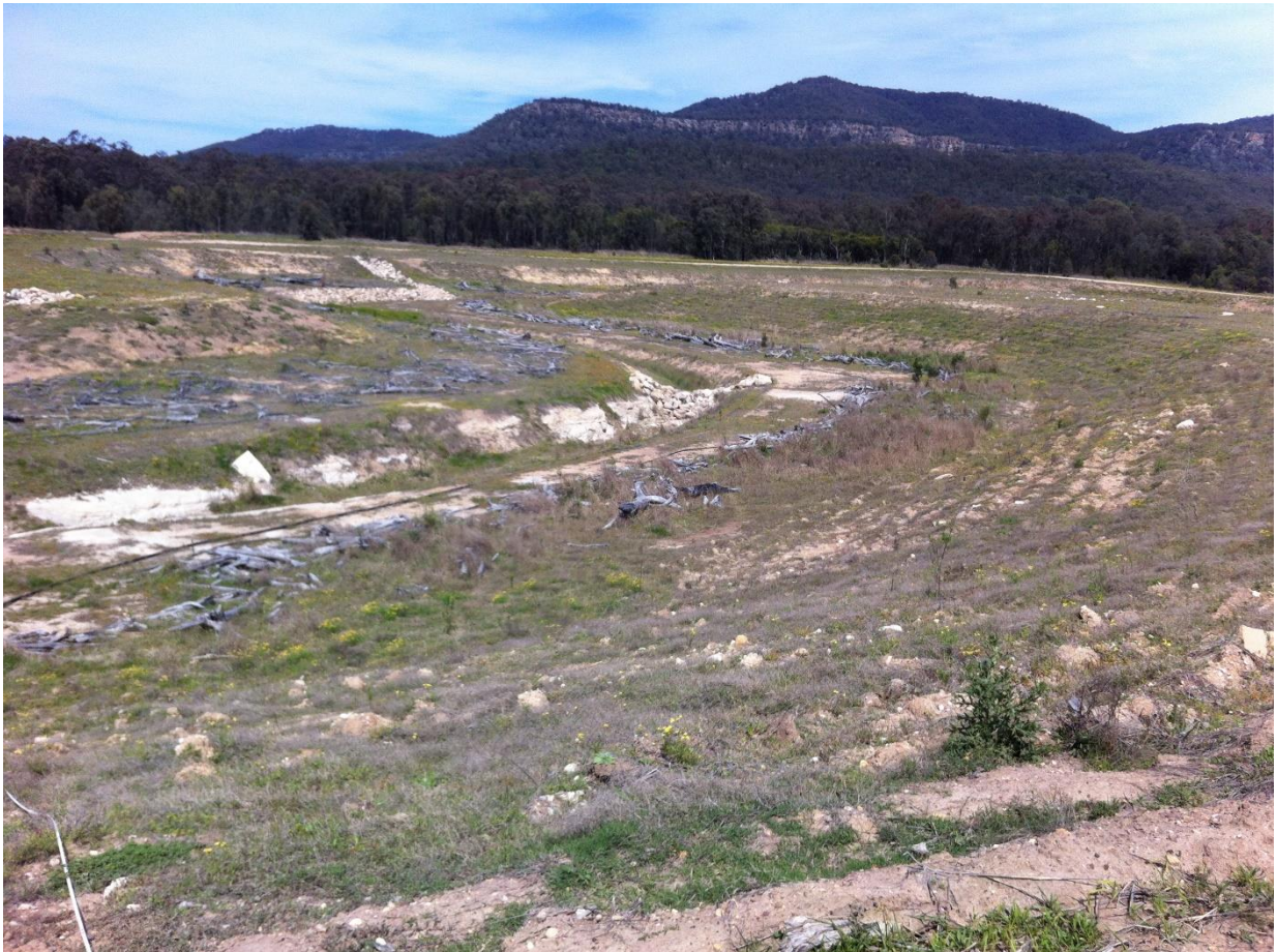
Plate 13: North Wambo Creek diversion near site 25R
