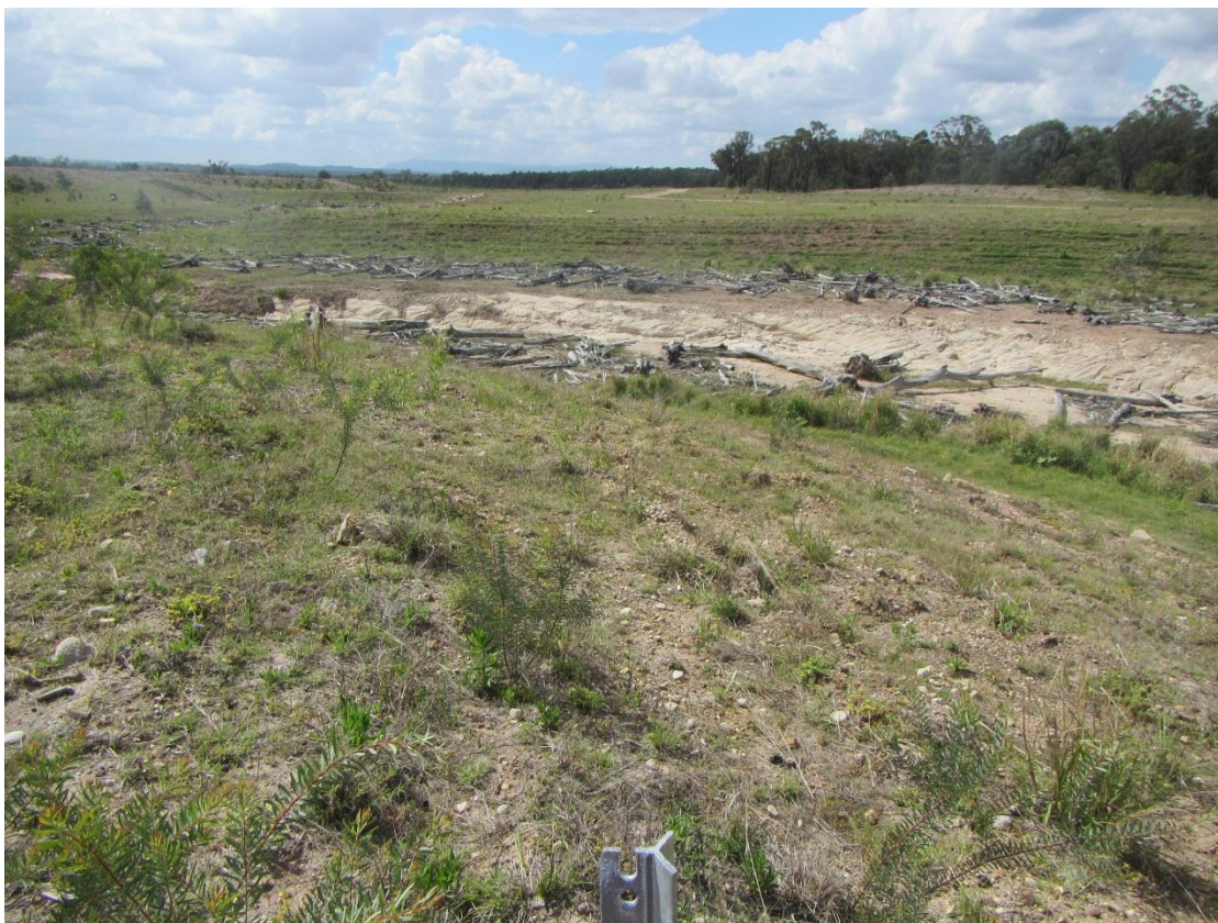
Figure 2-12. Improving woody vegetation establishment following light ripping of diversion batters
