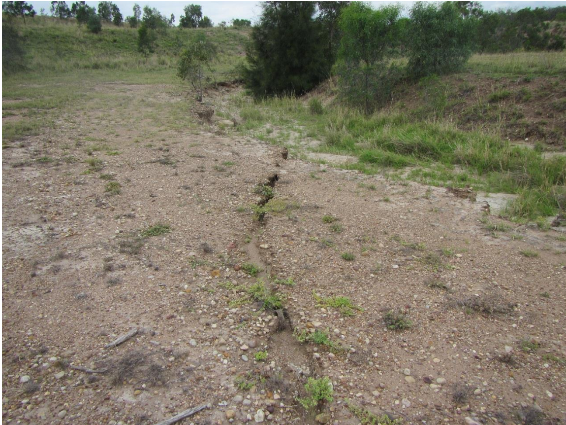
Figure 2-8. Cracking in inset floodplain over LW 11 in dispersive soils may lead to new tunnel and gully erosion
