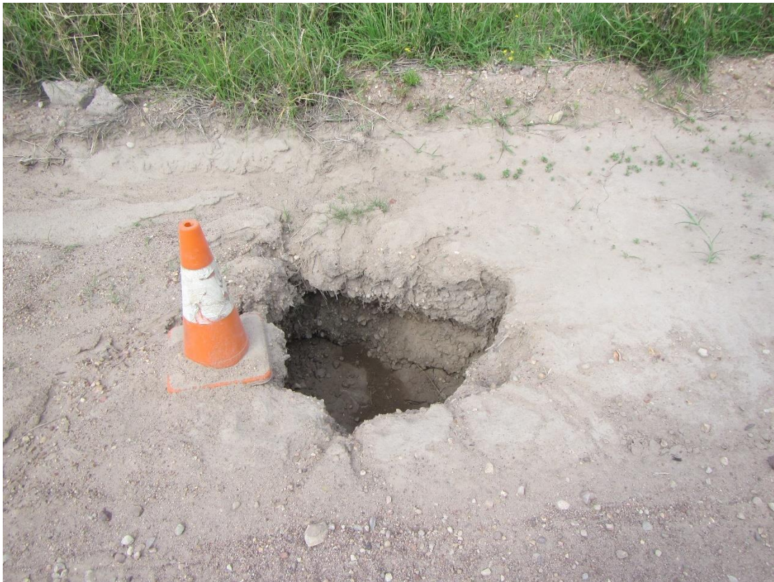
Figure 3-2 - Tunnelling over LW12/15 on track adjacent diversion
