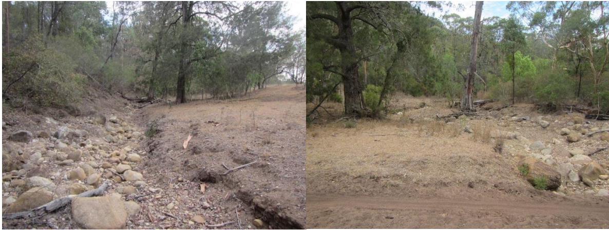
Figure 2-3. Partly confined North Wambo Creek, downstream of confluence of Spring and Chalkers Creeks
