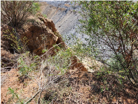
Existing erosion where tributary drops over highwall
