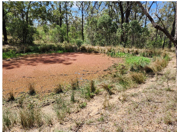
Small dam on edge of LW24 that is likely to be destabilised by subsidence
