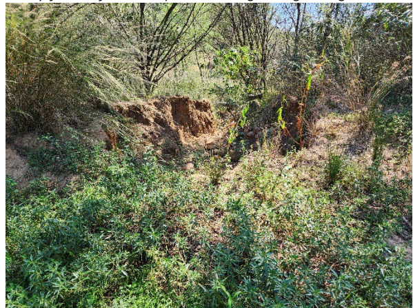
The embankment of the farm dam has already breached and may be subject to rapid failure in future flows.
