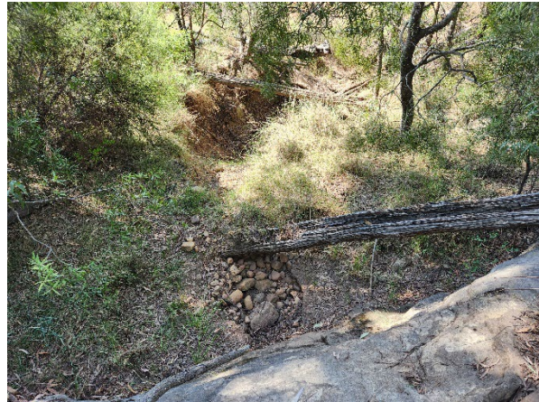
Headcut migration upstream in response to drop over highwall with bedrock control limiting extent
