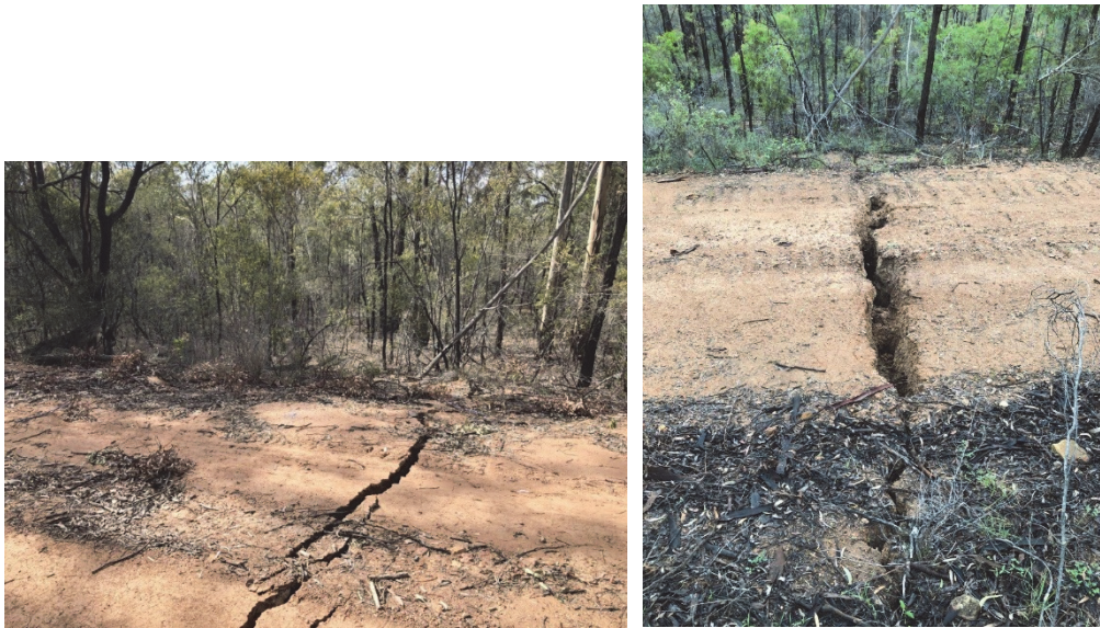
Fig. 4.11 Surface cracking along an access track above WYLW18 and WYLW19 (Source: WCPL)
