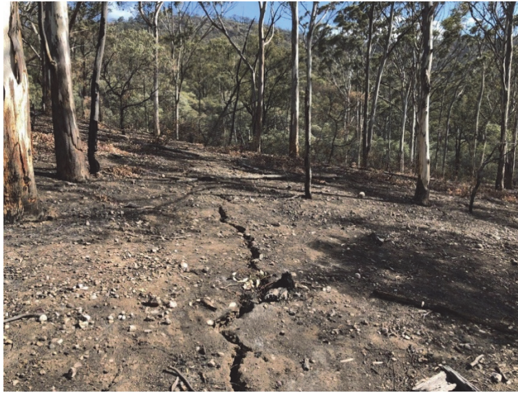
Fig. 4.10 Surface cracking on a steep slope above the south-western end of WYLW18
