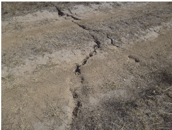
Fig. 4.6 Surface cracking along the access tracks above WYLW17
