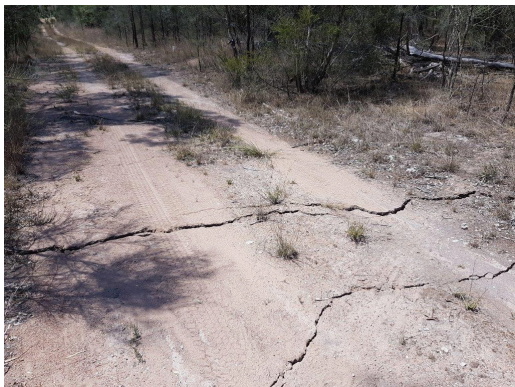
Fig. 4.8 Cracking and compression heaving along the tracks above WYLW12 (Source: WCPL)
