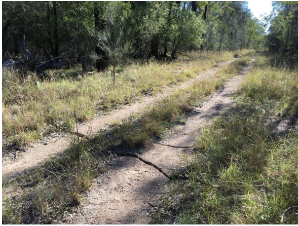
Fig. 4.12 Cracking along the access tracks above the central part of WYLW13 (Source: WCPL)
