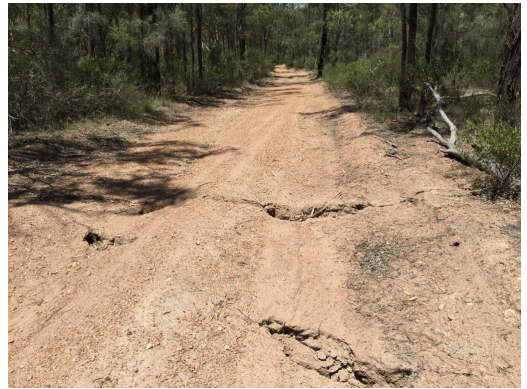
Fig. 4.7 Cracking along the fire trails above WYLW12 (Source: WCPL)
