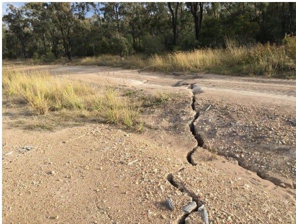
Fig. 4.11 Cracking above the north-eastern end of WYLW13 (Source: WCPL)
