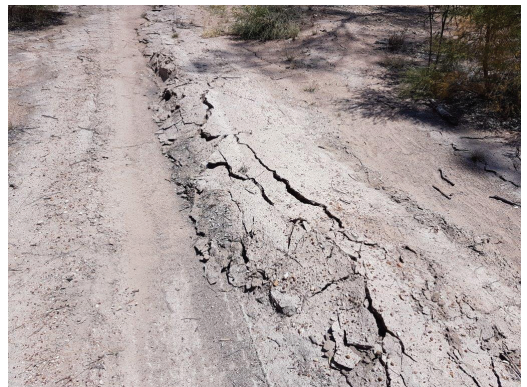
Fig. 4.8 Cracking and compression heaving along the tracks above WYLW12 (Source: WCPL)
