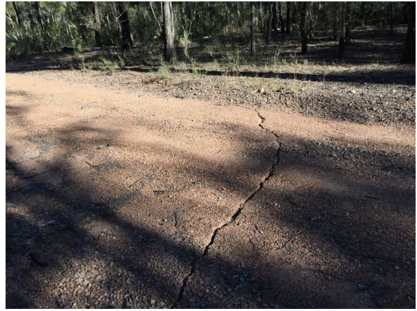
Fig. 4.12 Cracking along the access tracks above the central part of WYLW13 (Source: WCPL)
