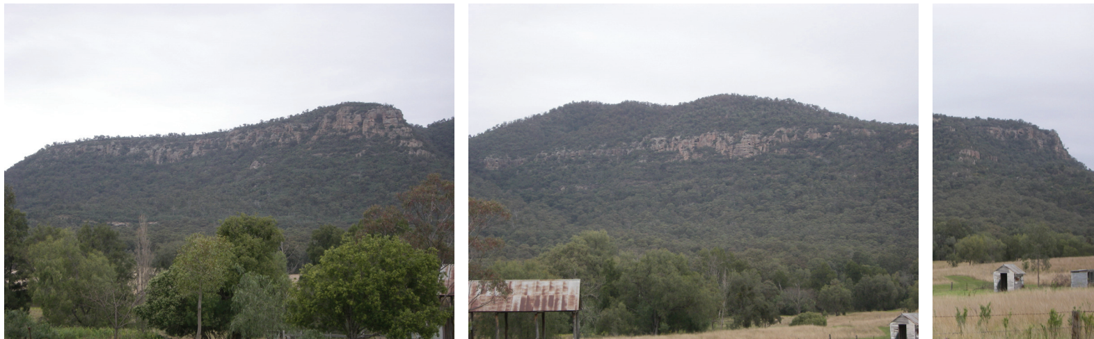
Fig. 5.13 Cliffs located south-west of the proposed WYLW21 to WYLW23 (P2929, P2930 and P2927)
