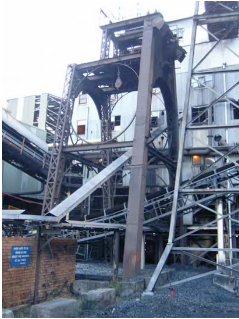
Plate 1 Shaft No. 1 Headframe
