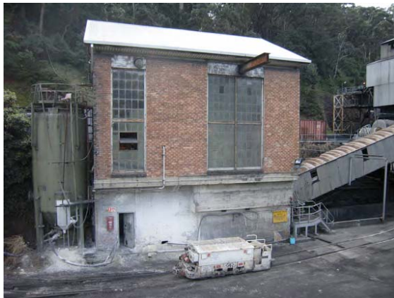
Plate 2 Drift Portal Winding House
