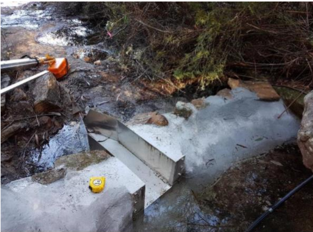
Typical "H flume" weir design and construction
