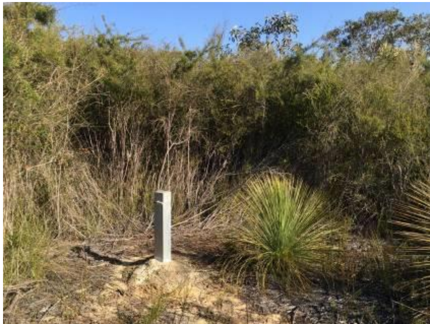
Photo of a typical groundwater bore installation within a swamp. Note vegetation re-establishing within the cleared area following construction.
