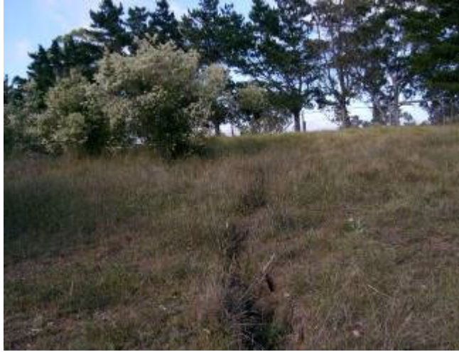
Fig. 4.15 Surface Tension Cracking along the Top of a Steep Slope
