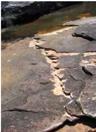
Fig. 4.17 Fracturing and Bedding Plane Slippage in Sandstone Bedrock in the Base of a Stream
