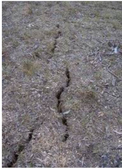
Fig. 4.16 Surface Tension Cracking along the Top of a Steep Slope
