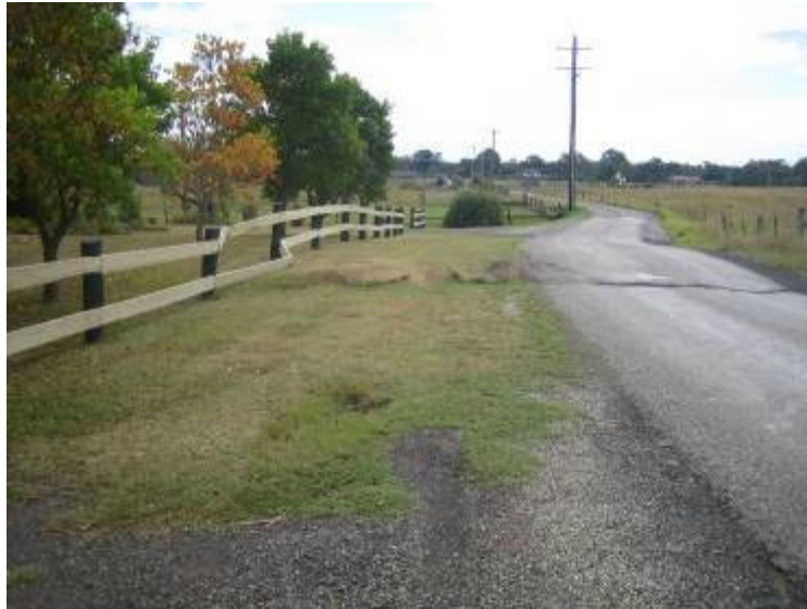
Fig. 4.12 Surface Compression Humping due to Low Angle Thrust Fault
