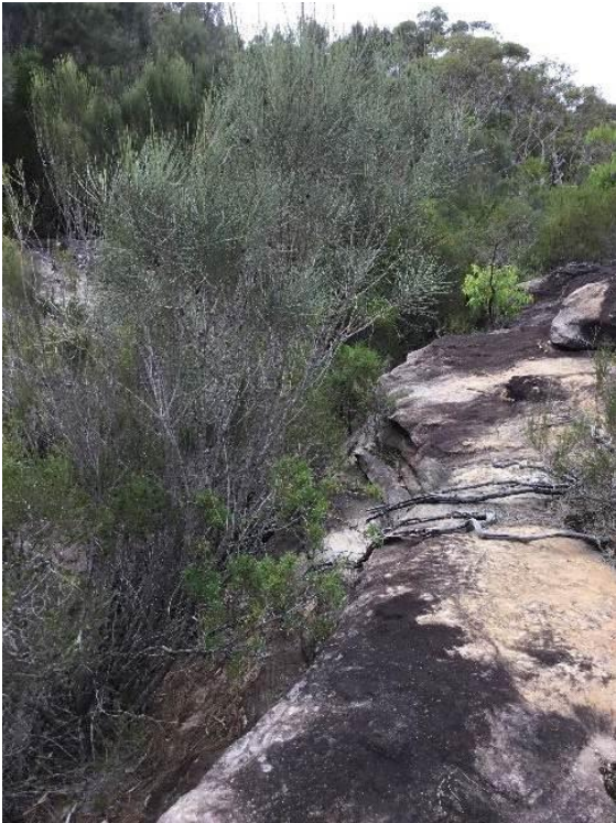
Photo P6 (Downstream)
