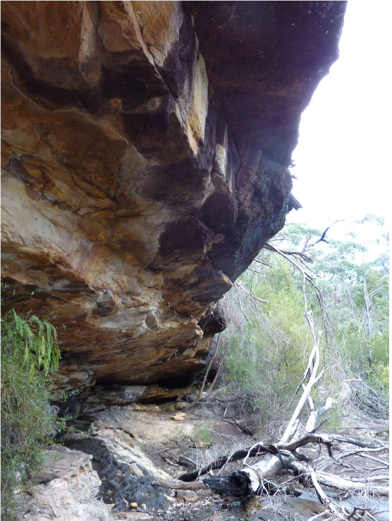
Photo C16-04 Overhang Looking Upstream
