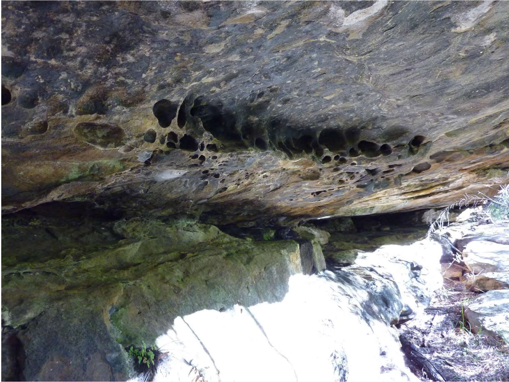
Photo C4-03 Eastern End Looking Upstream
