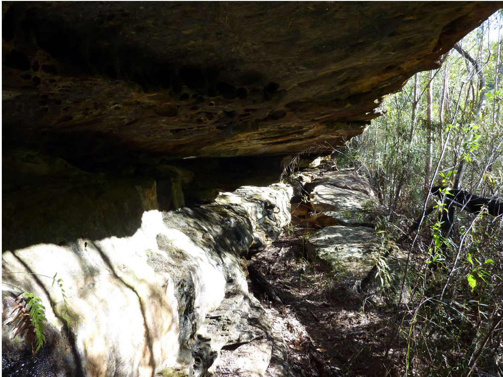
Photo C4-02 Eastern End Looking Upstream
