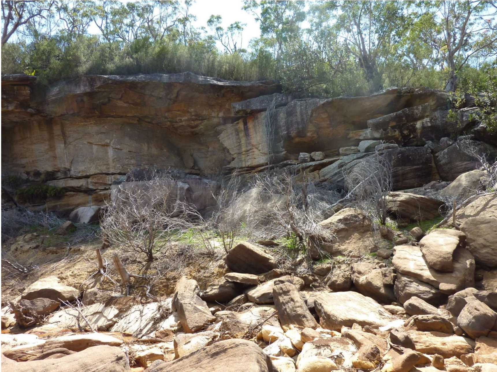
Photo C17-03 South Eastern End Looking North East
