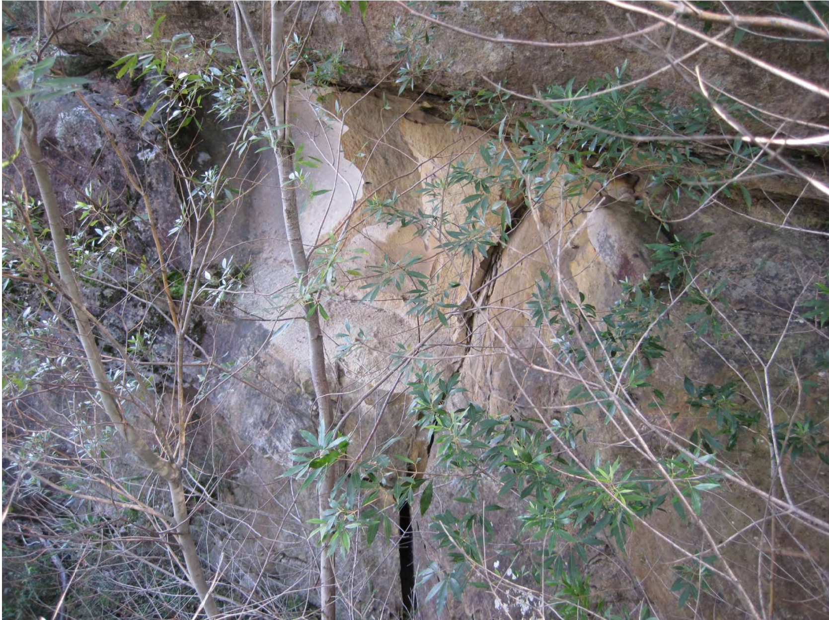
Photo C15-03 Eastern End – Existing Fracture in Rock
