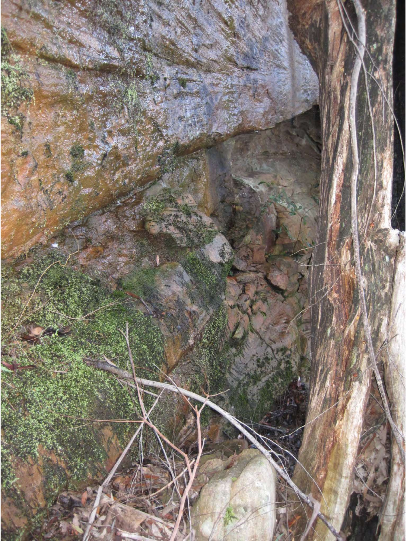
Photo C15-07 Western End Looking Downstream
