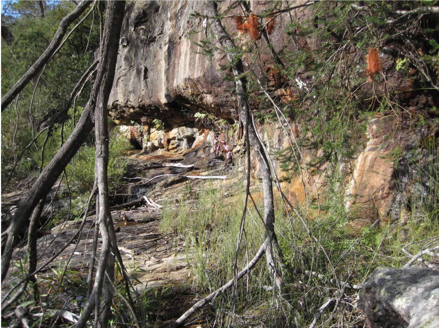
Photo C6A-06 Seepage Downstream from Cliff
