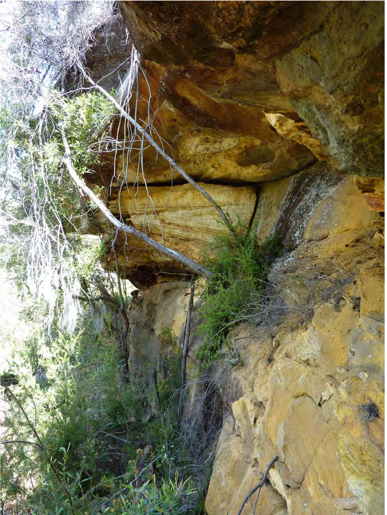
Photo C2-06 Northern end of main overhang
