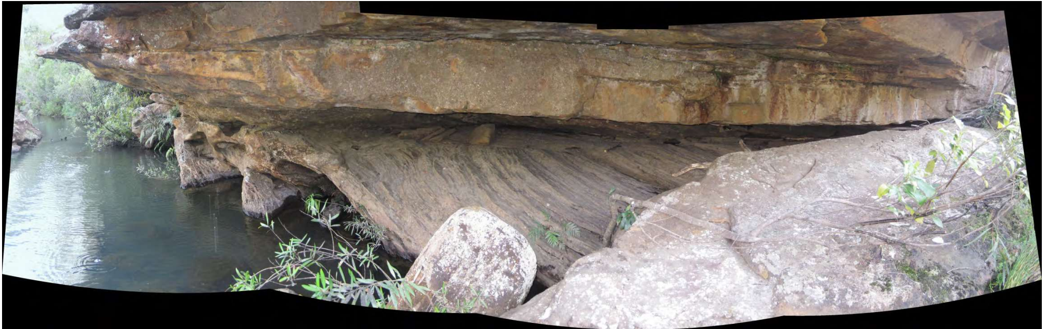
Photo C5-04 Overhang, height ~2.5m, depth ~7m, Looking North
