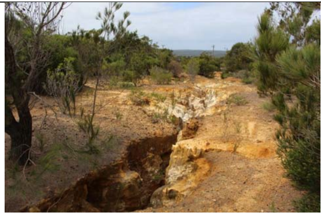
Subsidence monitoring line route heading east towards M1 Motorway.
