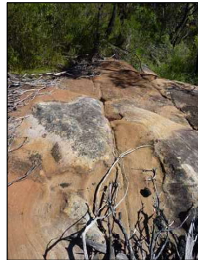
TB069-5 Joint with water
