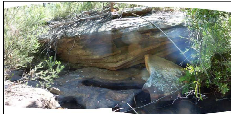
TA41-3 Overhang on east bank
