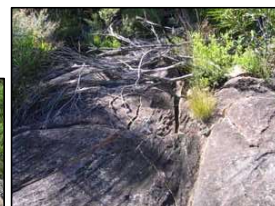
G1-5 Cracking in rockbar
