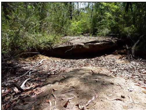
TB013-1 Dry creek bed looking Upstream
