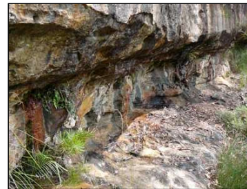
S-5 Iron staining at seepage
