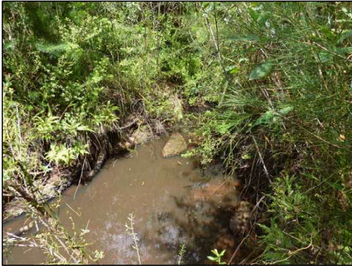
TB101-1 Downstream end of Pool TB-M looking Upstream
