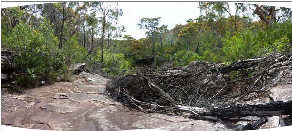
TB175-2 Upstream of Pool P looking Downstream
