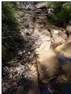
TA23-3 Joint downstream of Pool TA-I
