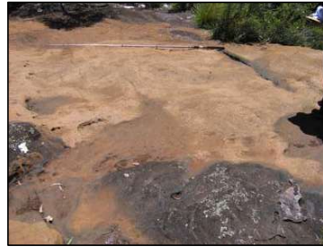
L-4 Joints across Rockbar K
