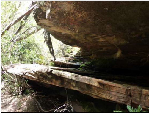
TB168-1 Overhang downstream of Pool TB-AN
