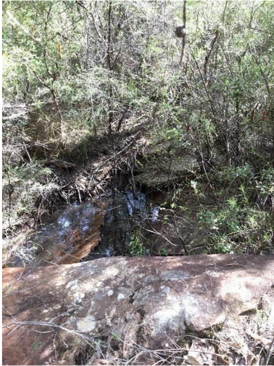
Photo S-East 2 (Downstream)
