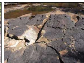
G1-6 Cracking in rockbar
