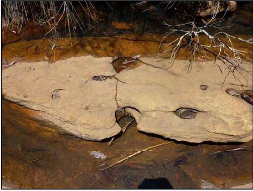
TA26-1 Cracking in rock
