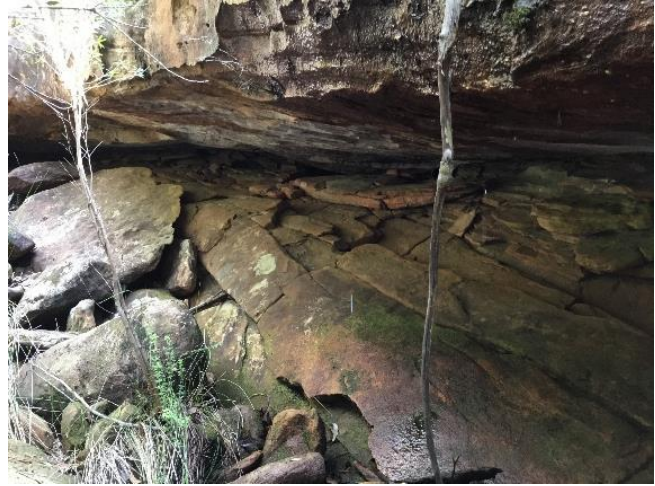
Photo F10 (Upstream 3)
