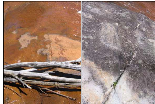
H-8 and H-9 Cracks in rockbar, 5mm wide, 5m apart.
