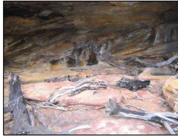
T-3 Iron stain at seepage, south east bank
