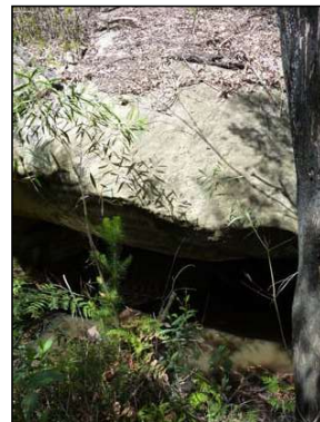
TB100-6 Overhang on southern bank
