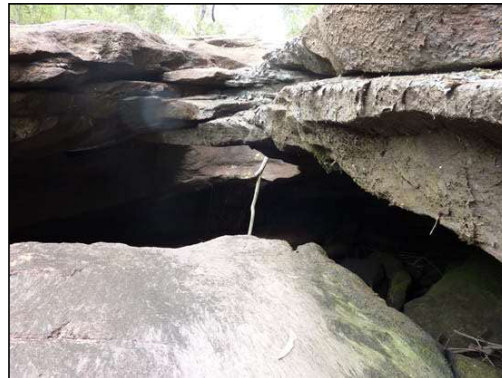
TB146-4 Pothole in overhang
