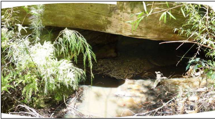
TB100-3 Near Downstream end of Pool TB-M looking toward southern bank
