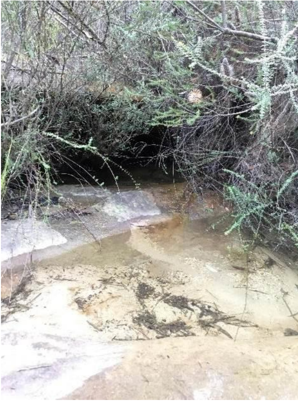
Photo F15 (Upstream)
