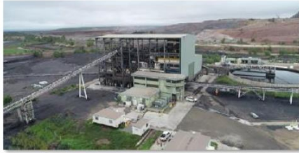
Coal Handling Prep Plant (CHPP) with successful history
