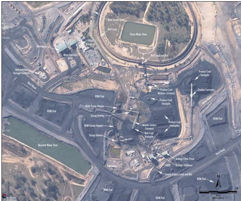
Figure 39. Central Infrastructure Aerial View
