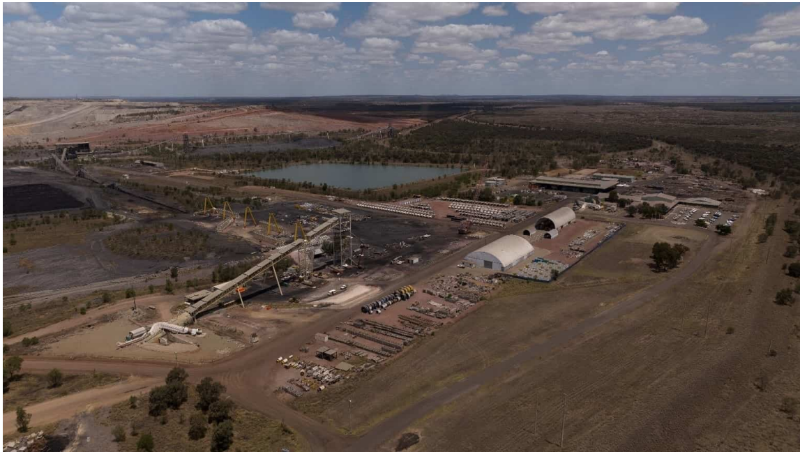
Figure 15-3. Centurion Surface Infrastructure
